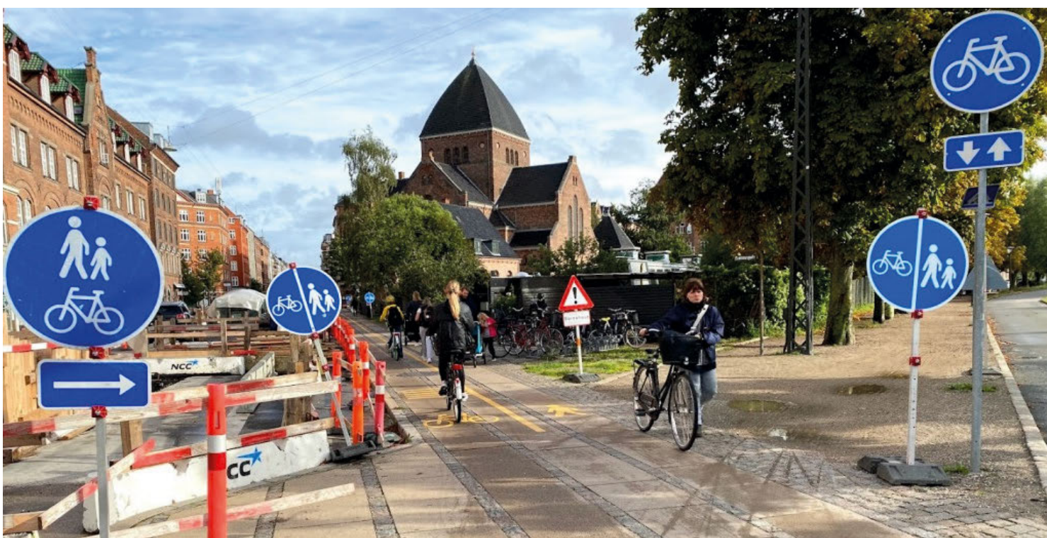
Roadworks, photo: City of Copenhagen
